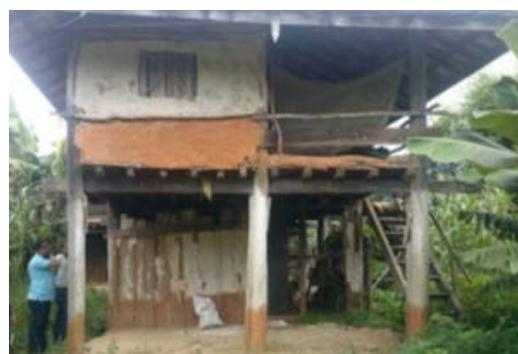
Figure 5: Typical timber frame structure
