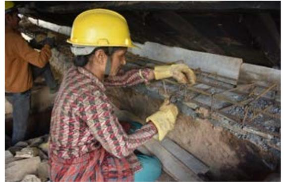
Figure 52: Participant constructing ring beam at ongoing training on strong back (Photo credit: UNOPS, Build Change, BBC Media Action Consortium)
