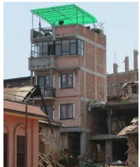
**Figure 7: Typical reinforced concrete frame building with masonry infill**
